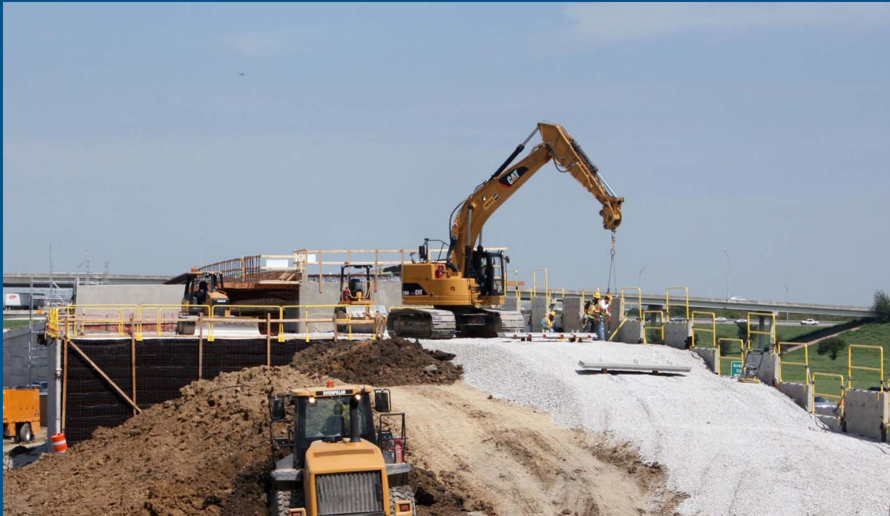
Wall: Mechanically Stabilized Earth (MSE) wall
